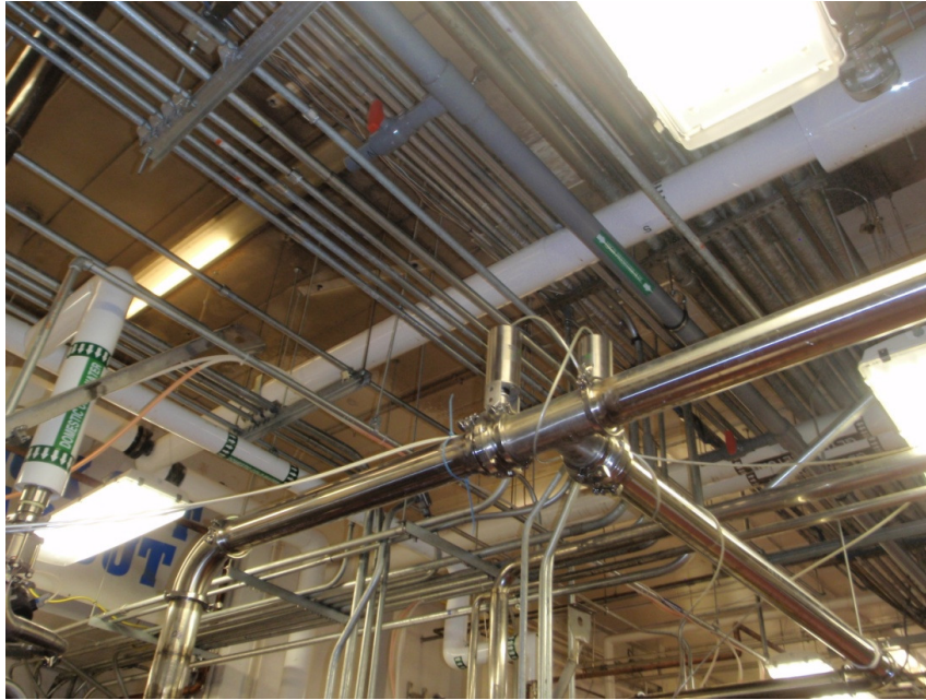
Freezer CIP Piping Modifications to Heat Exchanger
